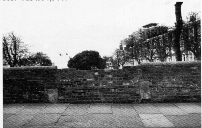
There is little evidence of any of the entrances on the surface. The Arklow Square entrance was between the two stone pillars. A change in the brickwork clearly shows where it was.
